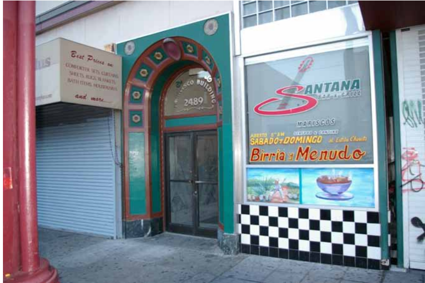
View looking northeast at the residential entrance Source: San Francisco Planning Department, September 2007
